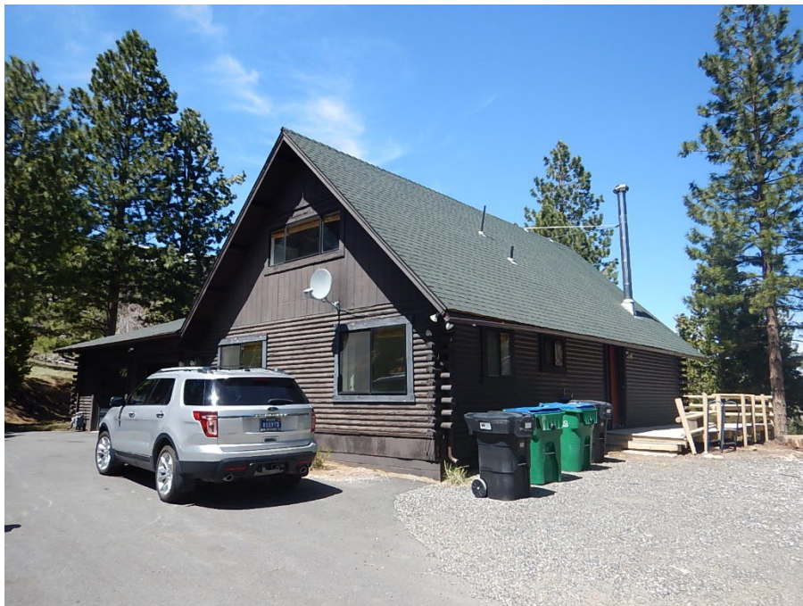
VIEW OF THE SUBJECT RESIDENCE FACING NORTHWESTERLY
