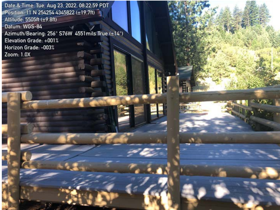
Looking west along the porch on the north side of the main residence.
