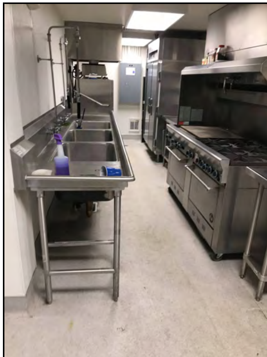
6 : View of kitchen in building interior.
