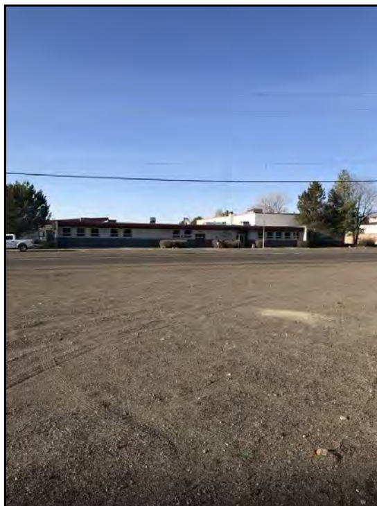
1 : View of northern portion of the Subject Property, facing south.
