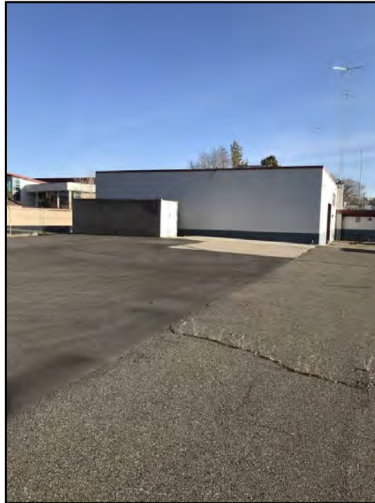
3 : View of southwestern portion of the Subject Property facing north,
