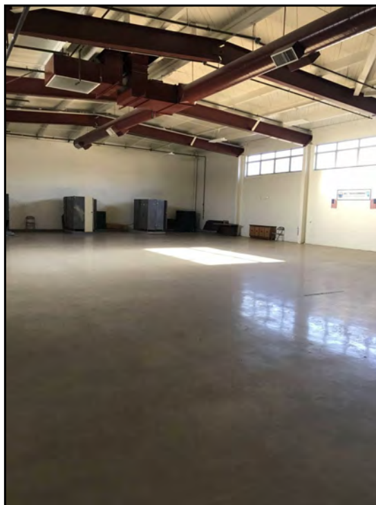
5 : View of gymnasium area and former indoor shooting range location.
