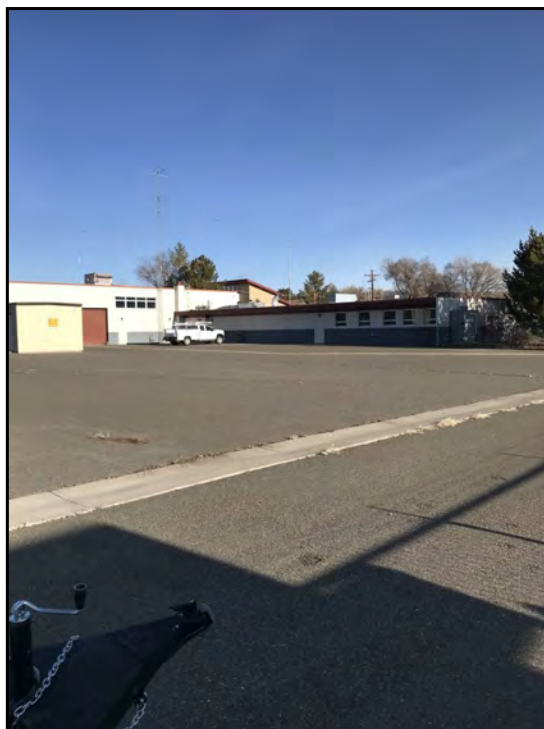
2 : View of southeastern portion of the Subject Property, facing northeast.
