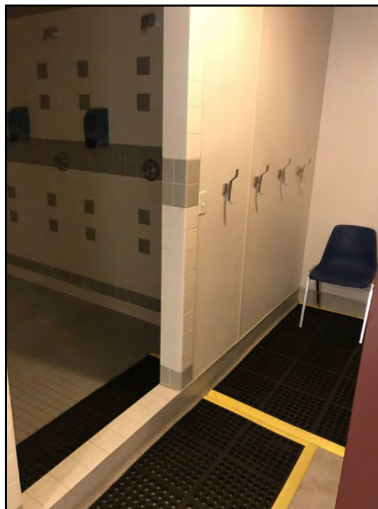
9 : View restroom and showers in building interior.
