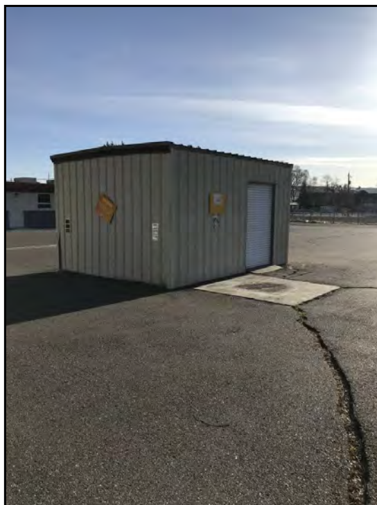
12 : materials building exterior in central portion of the Subject Property.
