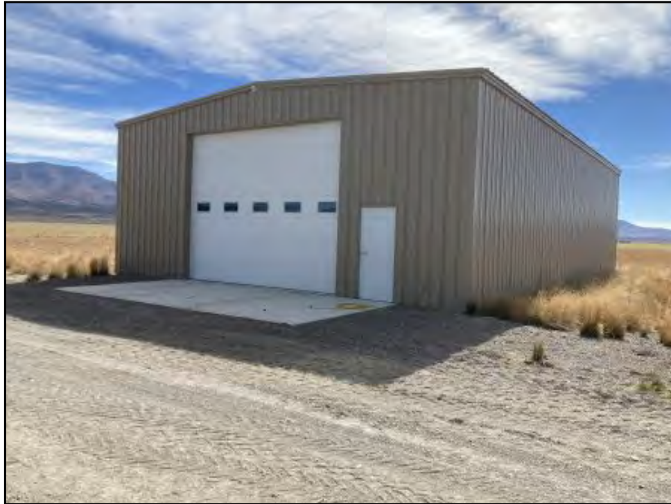
25 : View of the western portion of the Subject Property - shop building.
