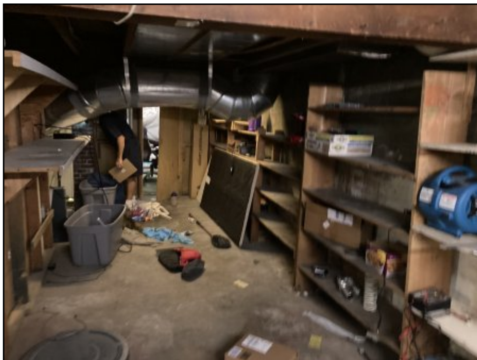
10 : View of the Subject Property interior.
