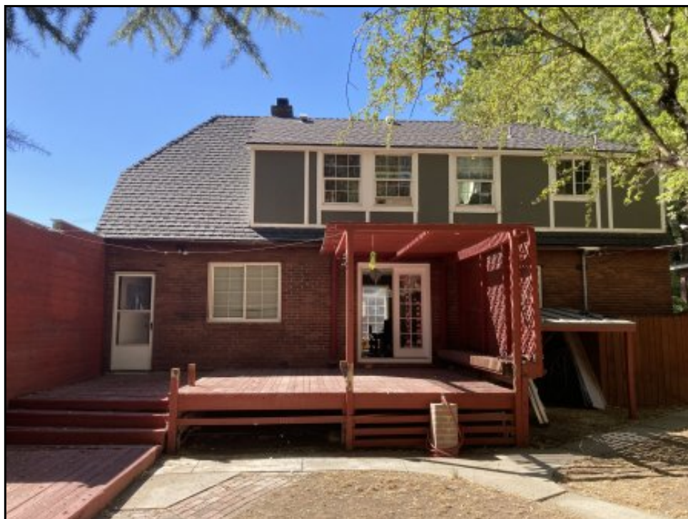
2 : View of the eastern Subject Property exterior, looking west.
