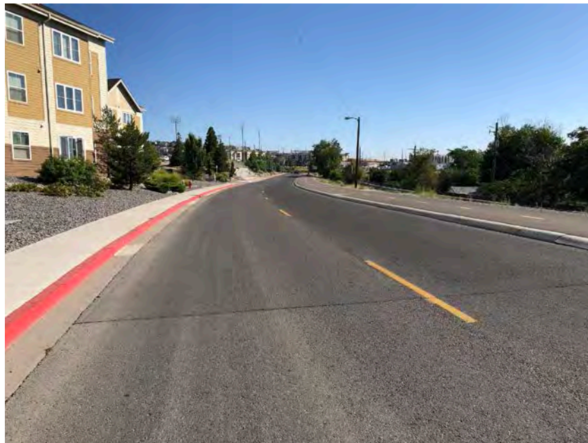
VIEW OF EVANS AVENUE FACING NORTHEAST FROM NEAR THE SUBJECT'S NORTHEAST PROPERTY CORNER
