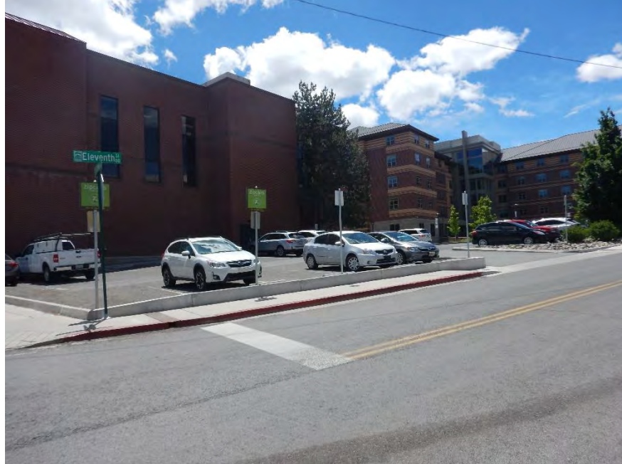
OVERALL VIEW OF SUBJECT FACING SOUTHWESTERLY FROM NORTH VIRGINIA STREET AND ELEVENTH STREET
