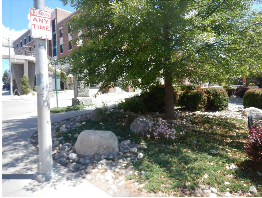
VIEW OF TEMPORARY CONSTRUCTION EASEMENT TCE-2 FACING NORTHEASTERLY FROM NORTH VIRGINIA STREET
