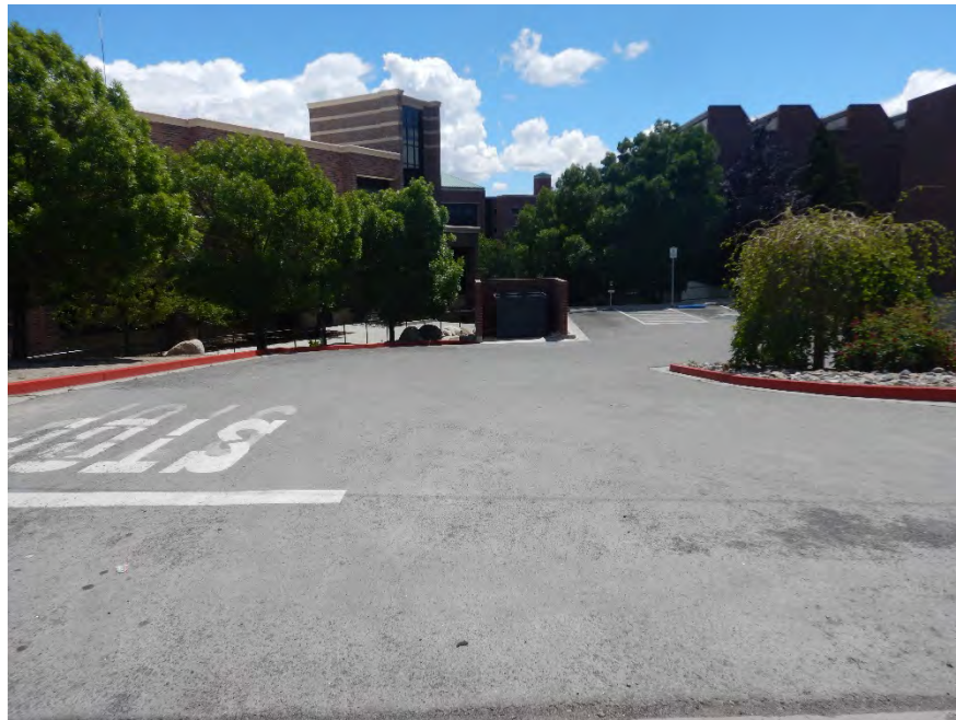
VIEW OF TEMPORARY CONSTRUCTION EASEMENT TCE-4 FACING EASTERLY FROM NORTH VIRGINIA STREET
