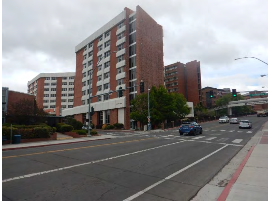
OVERALL VIEW OF SUBJECT PROPERTY FACING NORTHWESTERLY FROM NORTH VIRGINIA STREET
