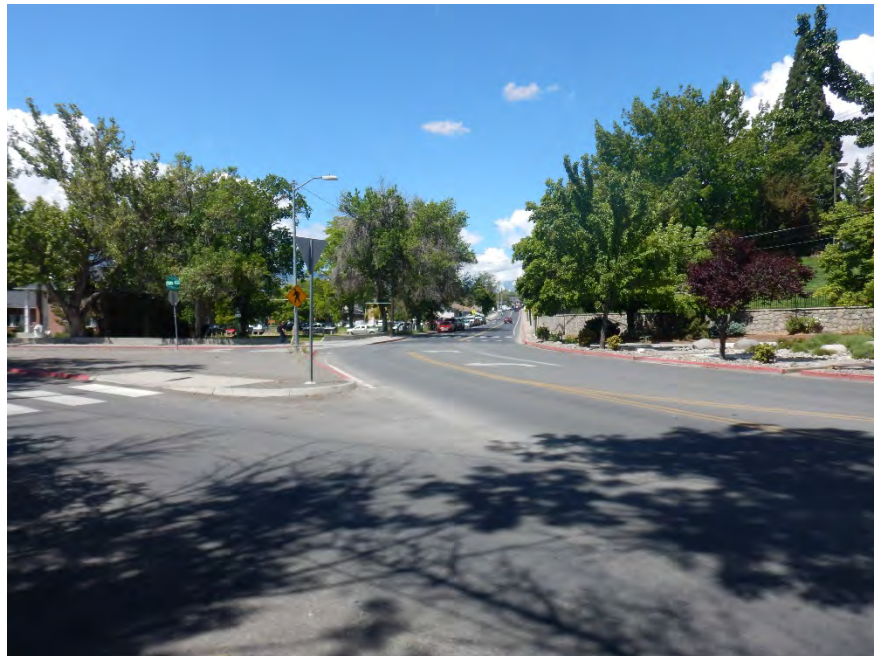
VIEW OF EAST NINTH STREET FACING WESTERLY FROM EVANS AVENUE
