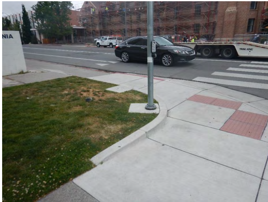
VIEW OF TEMPORARY CONSTRUCTION EASEMENT TCE 1 FACING NORTHEASTERLY FROM TENTH STREET
