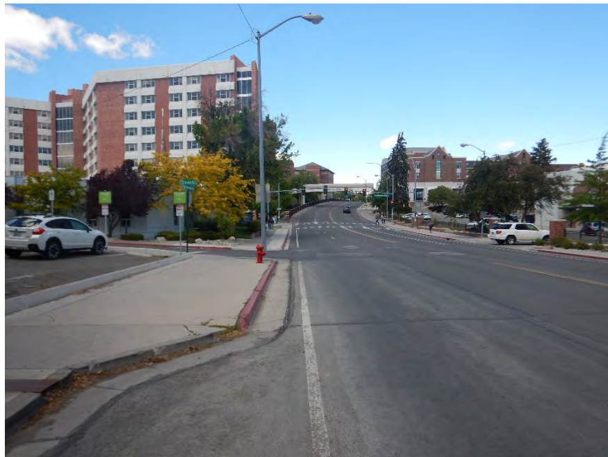
VIEW OF NORTH VIRGINIA STREET FACING NORTHERLY TOWARDS ELEVENTH STREET
