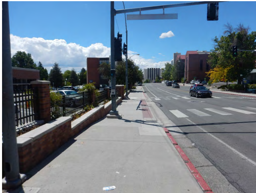
VIEW OF TEMPORARY CONSTRUCTION EASEMENT TCE-1 FACING SOUTHERLY AT THE INTERSECTION OF ARTEMESIA WAY
