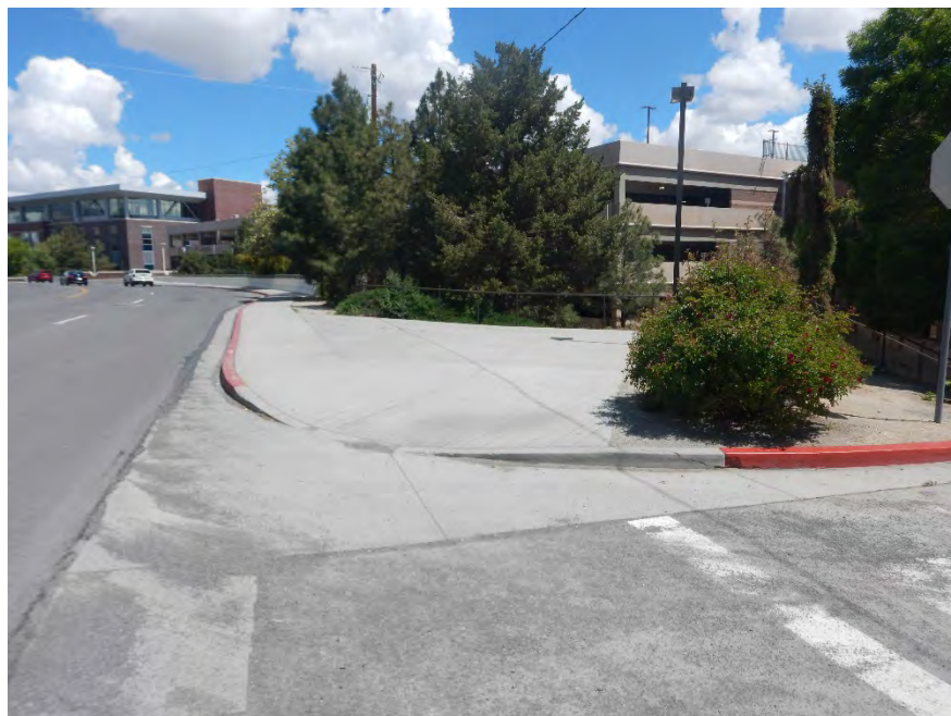
VIEW OF PERMANENT EASEMENT PE-3 FACING NORTHEASTERLY
