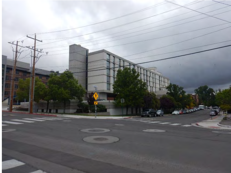
OVERALL VIEW OF SUBJECT PROPERTY FACING NORTHEASTERLY FROM TENTH STREET AND NORTH SIERRA STREET
