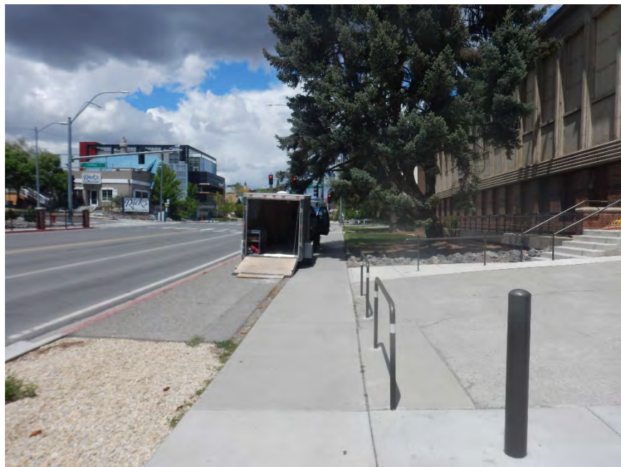
VIEW OF TEMPORARY CONSTRUCTION EASEMENT TCE-3 FACING NORTHERLY ALONG NORTH VIRGINIA STREET AT COLLAGE DRIVE
