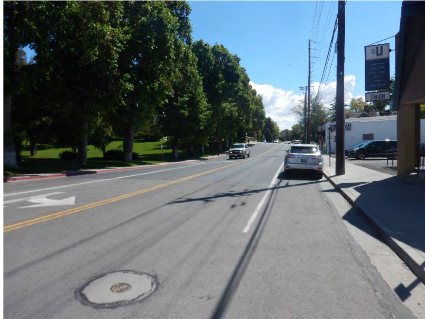
VIEW OF EAST NINTH STREET FACING EASTERLY FROM NORTH VIRGINIA STREET
