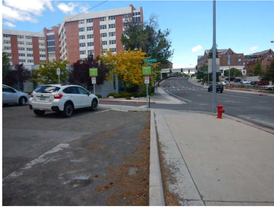
VIEW OF TEMPORARY CONSTRUCTION EASEMENT FACING NORTHERLY ALONG NORTH VIRGINIA STREET
