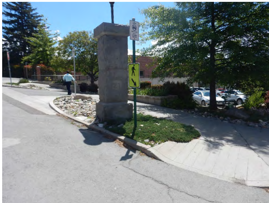
VIEW OF TEMPORARY CONSTRUCTION EASEMENT TCE-2 FACING SOUTHEASTERLY FROM NORTH VIRGINIA STREET
