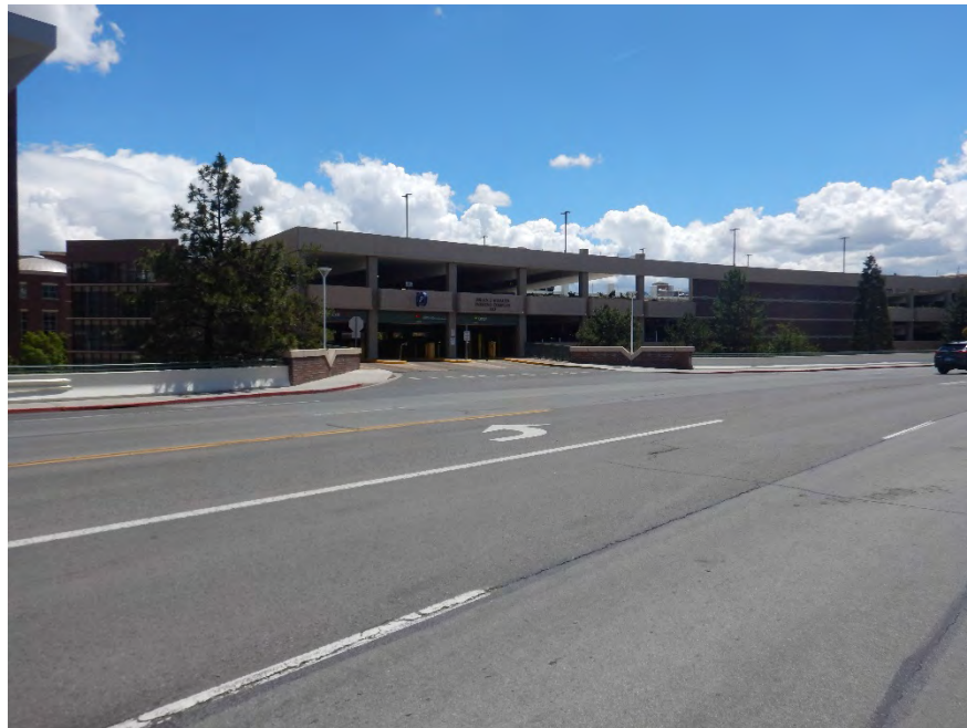
VIEW OF TEMPORARY CONSTRUCTION EASEMENT TCE-5 FACING SOUTHEASTERLY FROM NORTH VIRGINIA STREET
