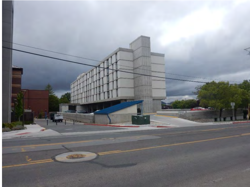
VIEW OF SUBJECT PROPERTY FACING SOUTHEASTERLY FROM NORTH SIERRA STREET
