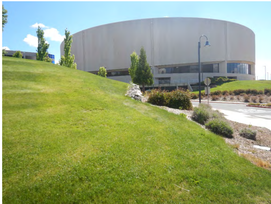
VIEW OF TEMPORARY CONSTRUCTION EASEMENT TCE-6 FACING SOUTHEASTERLY FROM NORTH VIRGINIA STREET
