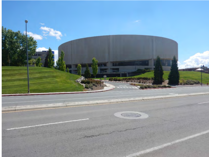
VIEW OF RIGHT-OF-WAY ACQUISITION 2 FACING SOUTHEASTERLY FROM NORTH VIRGINIA STREET
