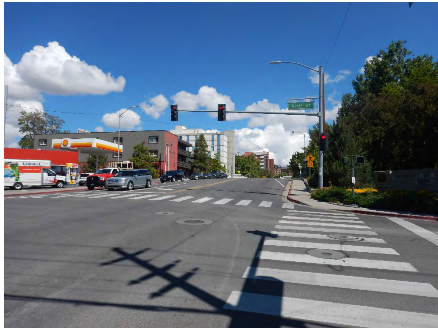
VIEW OF NORTH VIRGINIA STREET FACING NORTHERLY FROM NINTH STREET
