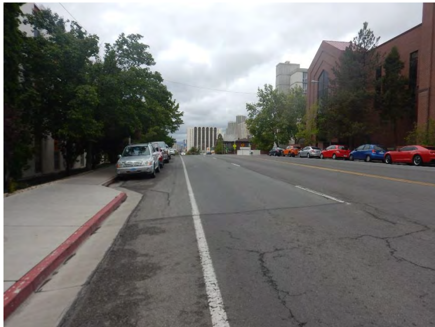
VIEW OF NORTH VIRGINIA STREET FACING IN A SOUTHERLY DIRECTION FROM ELEVENTH STREET
