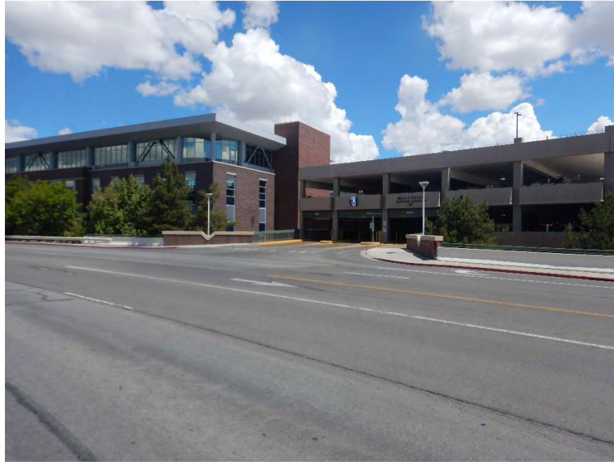
VIEW OF TEMPORARY CONSTRUCTION EASEMENT TCE-5 FACING NORTHEASTERLY FROM NORTH VIRGINIA STREET
