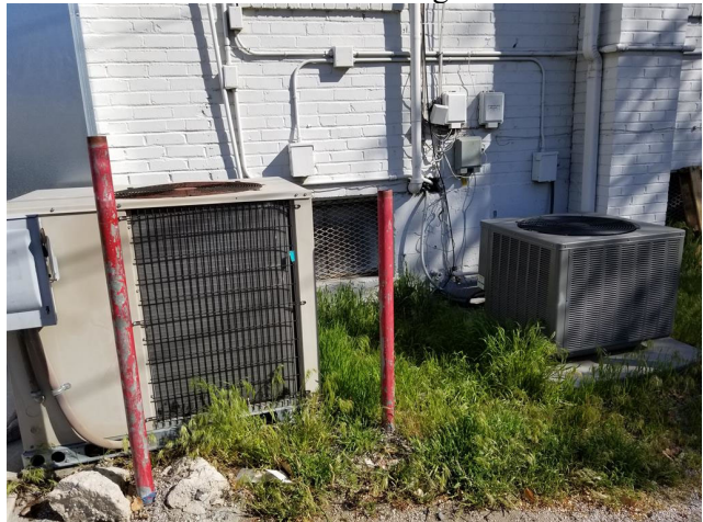
Exterior View – south side of building
