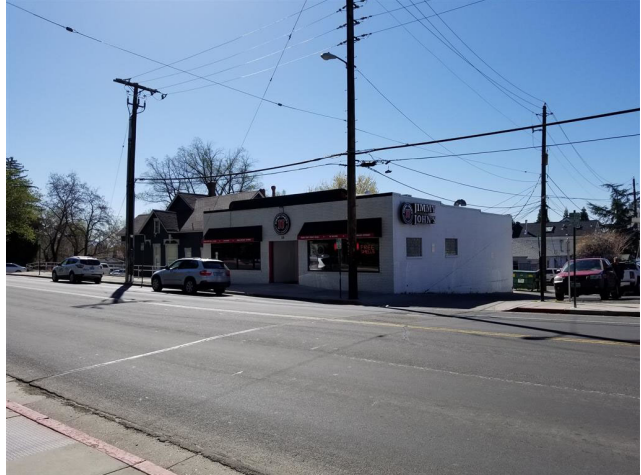
Exterior View looking southeast
