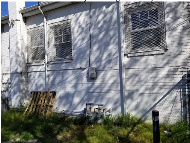
Exterior View – south side of building
