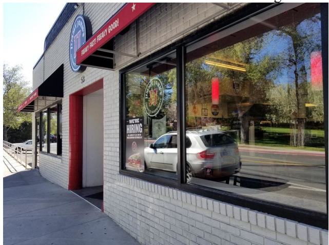
Exterior View – north side fronting 9 th Street
