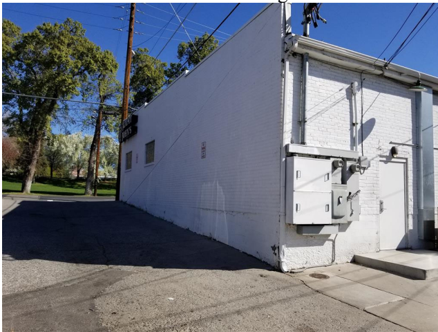
Exterior View looking northeast
