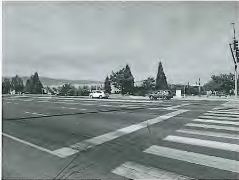
VIEW OF MILL AT MCCARRAN INDUSTRIAL FLEX COMPLEX FACING SOUTHWESTERLY FROM MILL STREET AND MCCARRAN BOULEVARD
