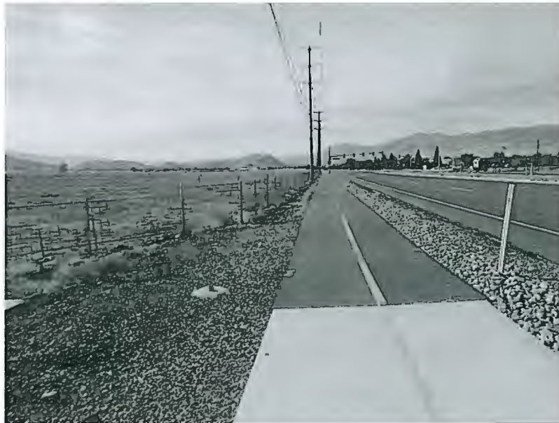
VIEW OF BICYCLE PATH ABUTTING SUBJECT'S WESTERLY PROPERTY LINE FACING SOUTHERLY ALONG SOUTH MCCARRAN BOULEVARD
