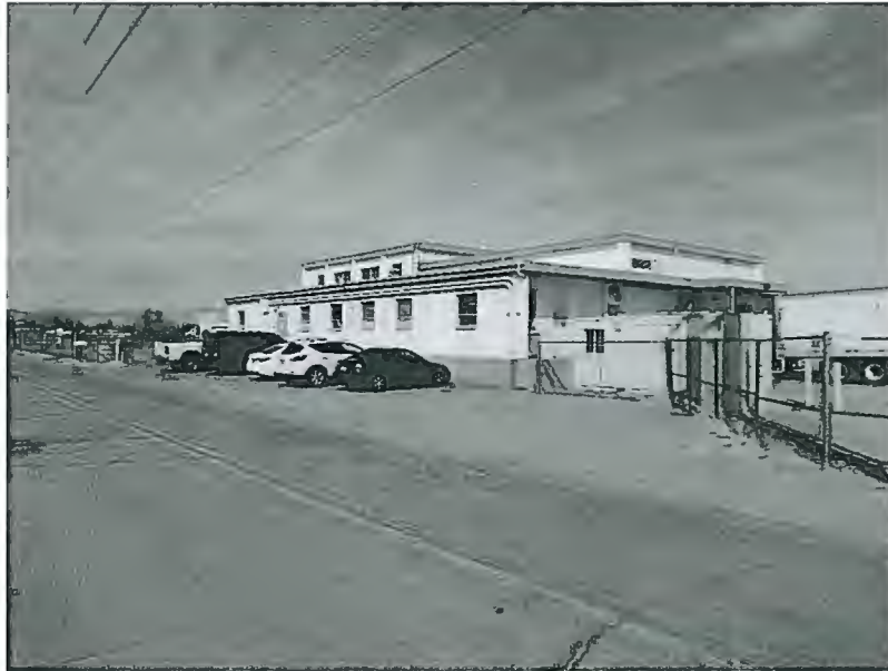
VIEW OF WOLF PACK MEATS, LOCATED ON THE NORTH SIDE OF CLEAN WATER WAY AND TO THE NORTH THE SUBJECT PROPERTY
