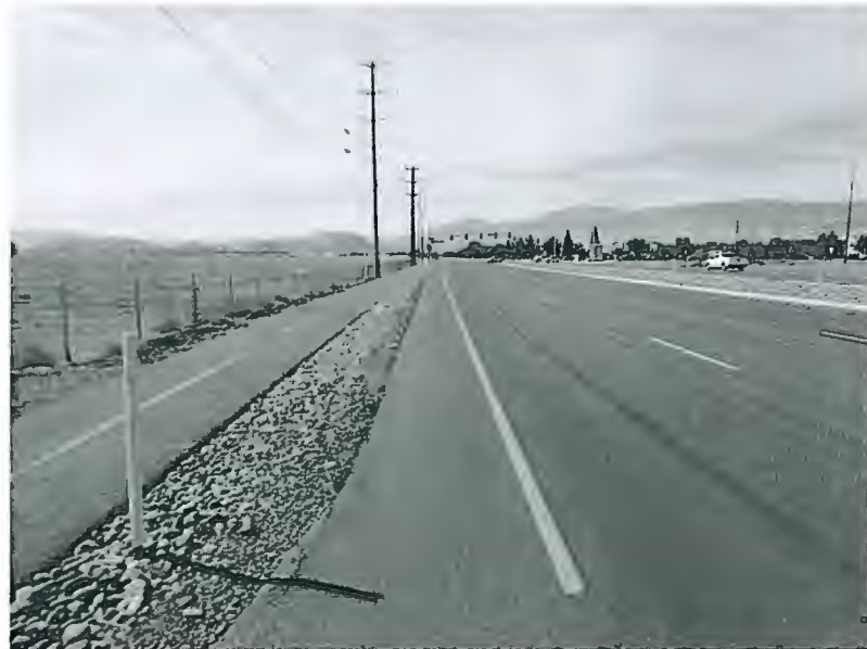
VIEW OF SOUTH MCCARRAN BOULEVARD FACING SOUTHERLY FROM CLEAN WATER WAY
