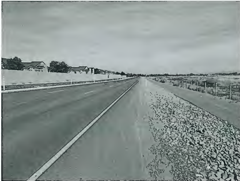
VIEW OF SOUTH MCCARRAN BOULEVARD FACING NORTHERLY FROM NEAR THE SOUTH PROPERTY LINE OF THE SUBJECT
