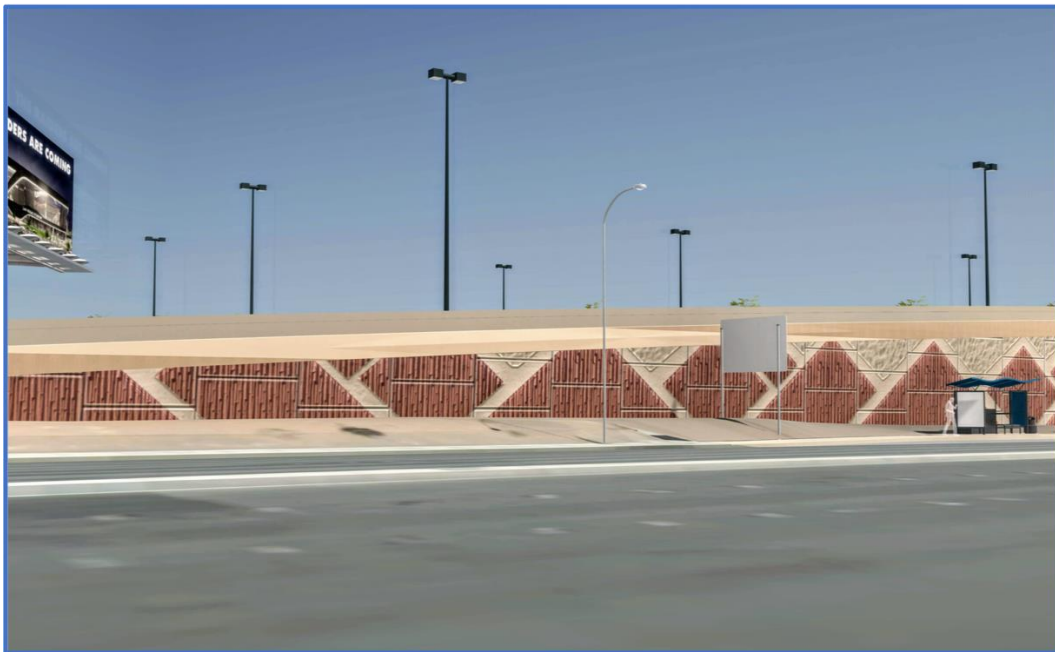
Figure 11. Tropicana Ave. EB Facing Northeast with Elevated Roadway (Image source: Clark County)
