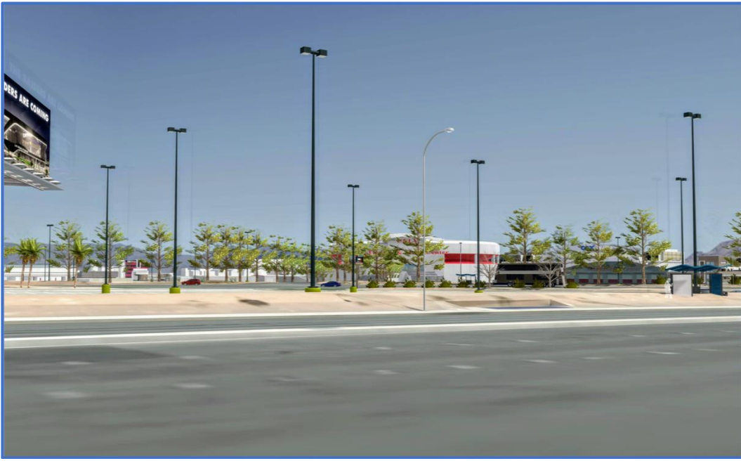
Figure 10. Tropicana Ave. EB Facing Northeast Current View (Image source: Clark County)
