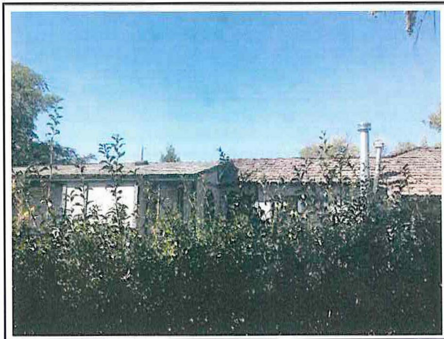
Photograph 13: View of the north-adjointing residence.
