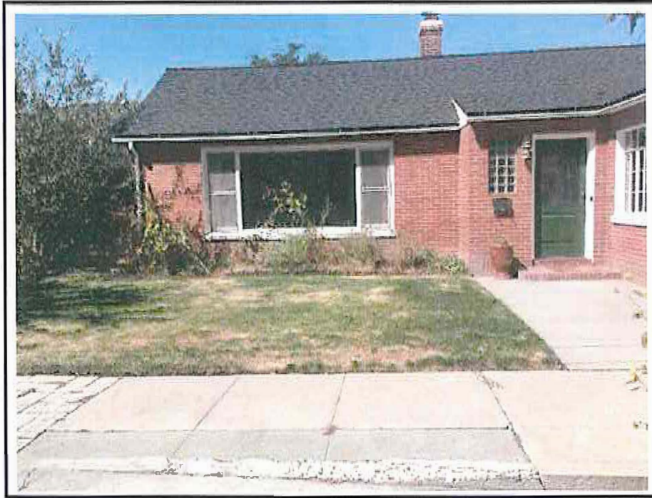
Photograph 1: Central portion of the Subject Property, looking northwest.
