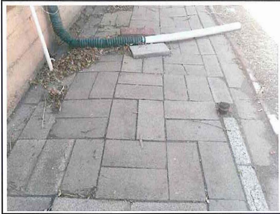
Photograph 11: View of the heating oil UST fill pipe and pavers covering the UST area along the northeastern exterior of the Subject Property building.
