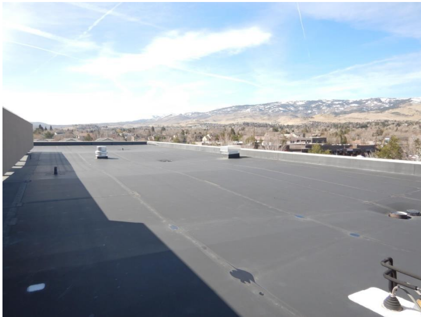
VIEW OF THE ROOF
