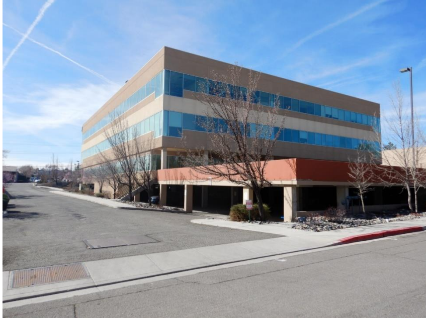
VIEW OF THE SUBJECT FACING SOUTHWEST FROM ISBELL ROAD
