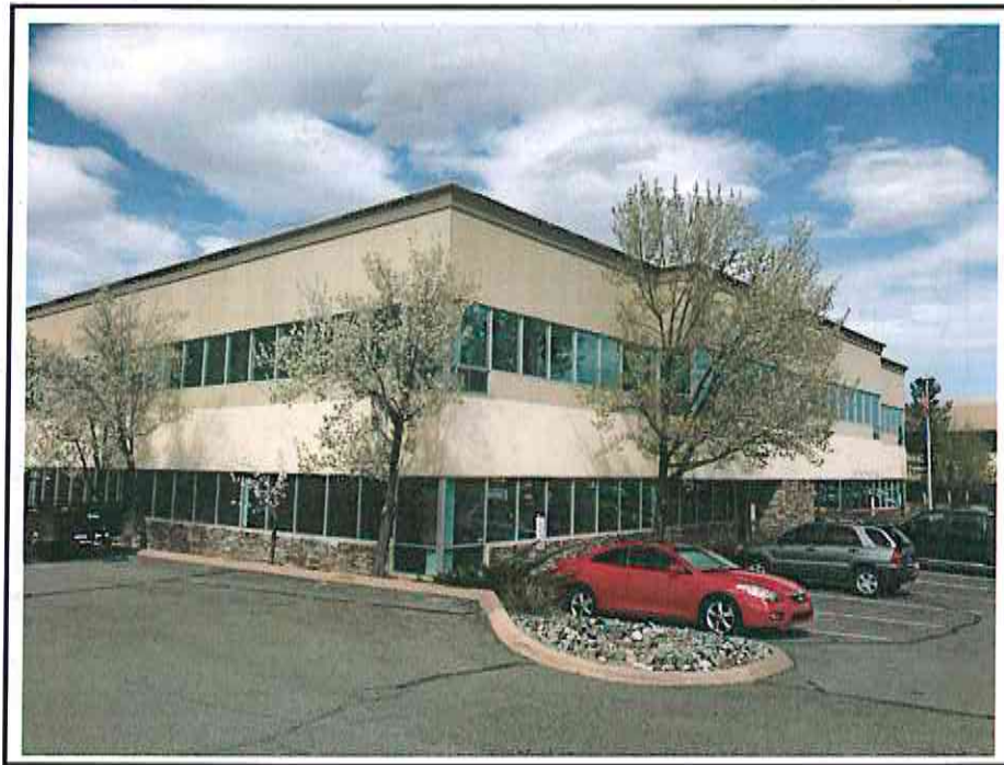
Photograph 7: View of the commercial offices located east of the Subject Property.
