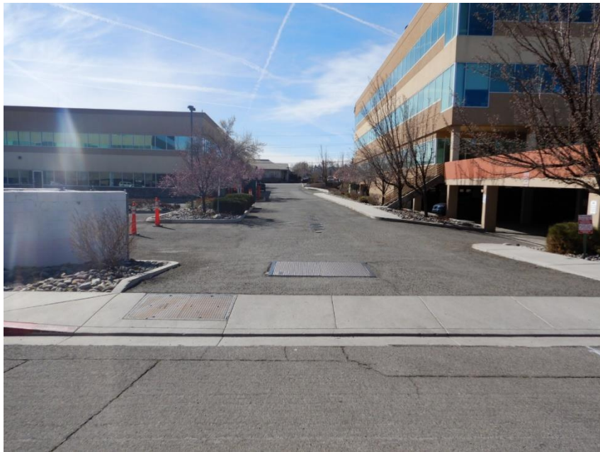
VIEW OF ACCESS ROAD ON EAST SIDE OF BUILDING
