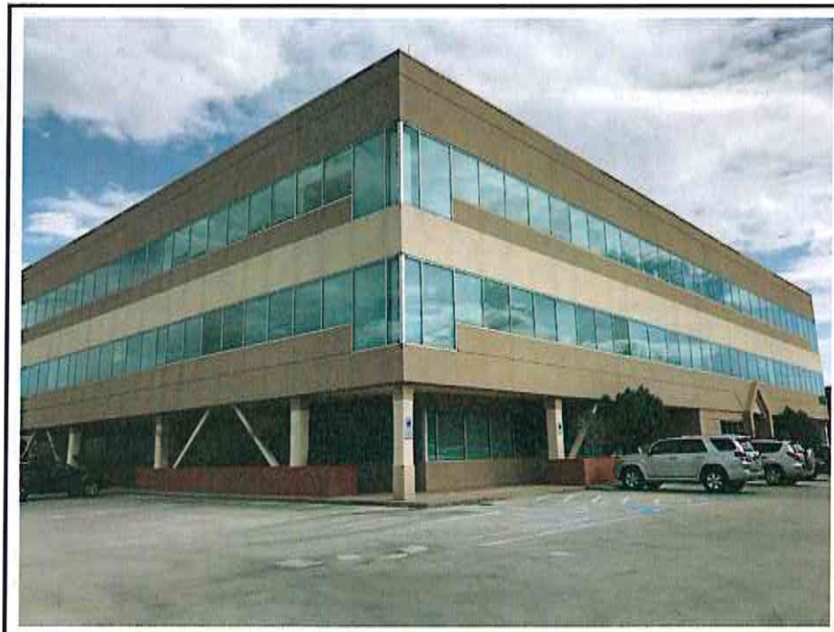
Photograph 2: Rear view of the Subject Property, looking south.
