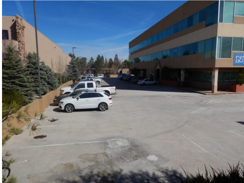
VIEW OF THE FIRST FLOOR PARKING
