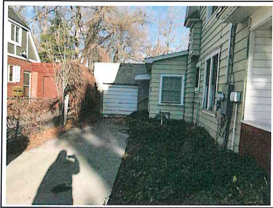
Photograph 3: View of the northern portion of the Subject Property.
