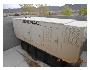
13. Photograph of backup generator taken from above edge of block wall in north corner of property. Generator is sitting atop a steel secondary containment structure, which is above a concrete slab. Minor fuel staining was noted on the slab.
