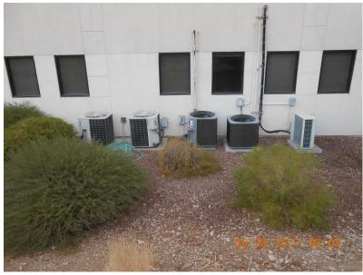
9. Air conditioning equipment on the south side of the building. There were no signs of any damage or stains on pads.
